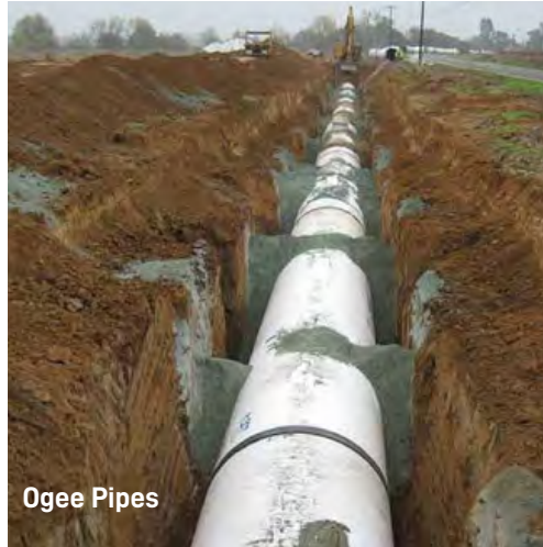
Spigot & Socket with Rigid Joint Pipes
